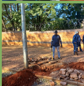
New cable & 3 phase meter installation at Kruger Str in Mokopane
