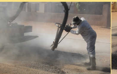
Patching of potholes at Molalaggori str in Mahwelereng
