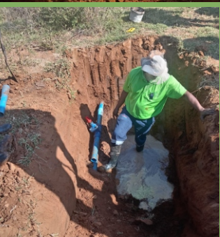
Pipe burst maintenance and replacement at Makekeng Village in Bakenberg Cluster
