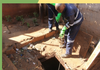
Unblocking of sewer line at Zone 1 in Mahwelereng
